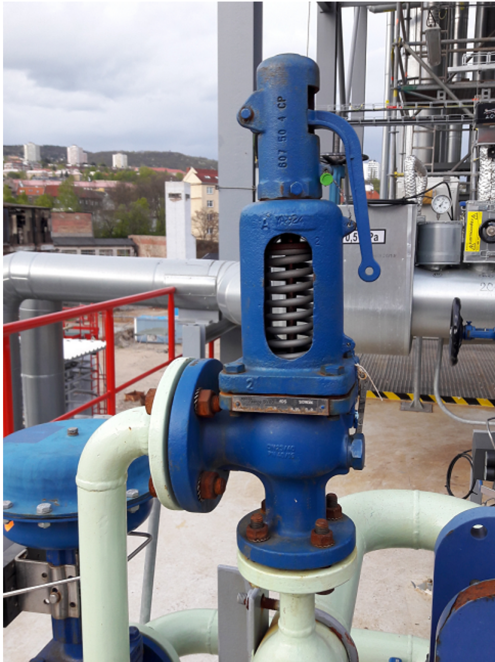
A pressure relief valve. Image source: Wikipedia
