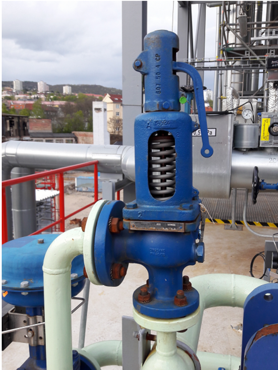
A pressure relief valve. Image source: Wikipedia
