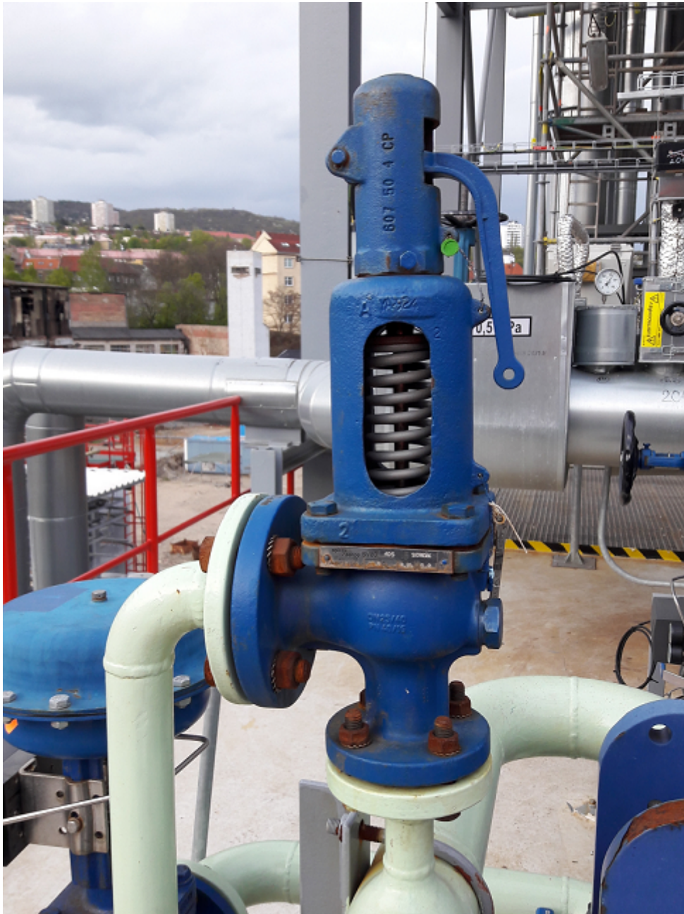
A pressure relief valve. Image source: Wikipedia
